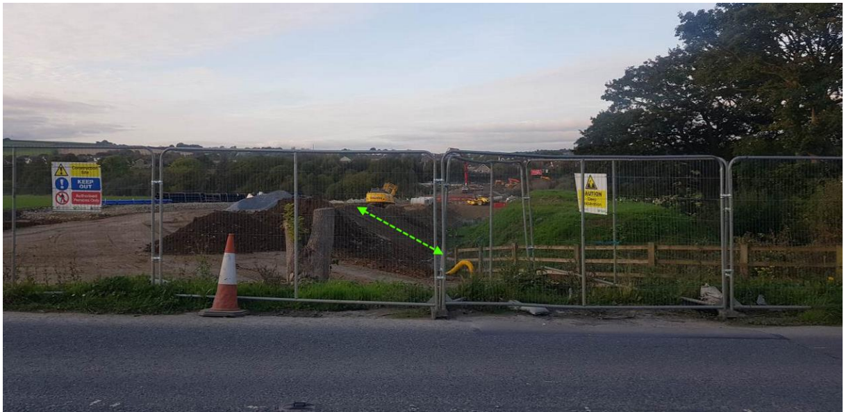
Figure 6: Embankments at site
